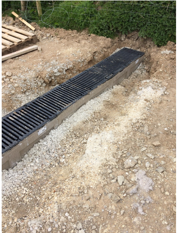
Track cross drain in construction, designed to take heavy machinery
