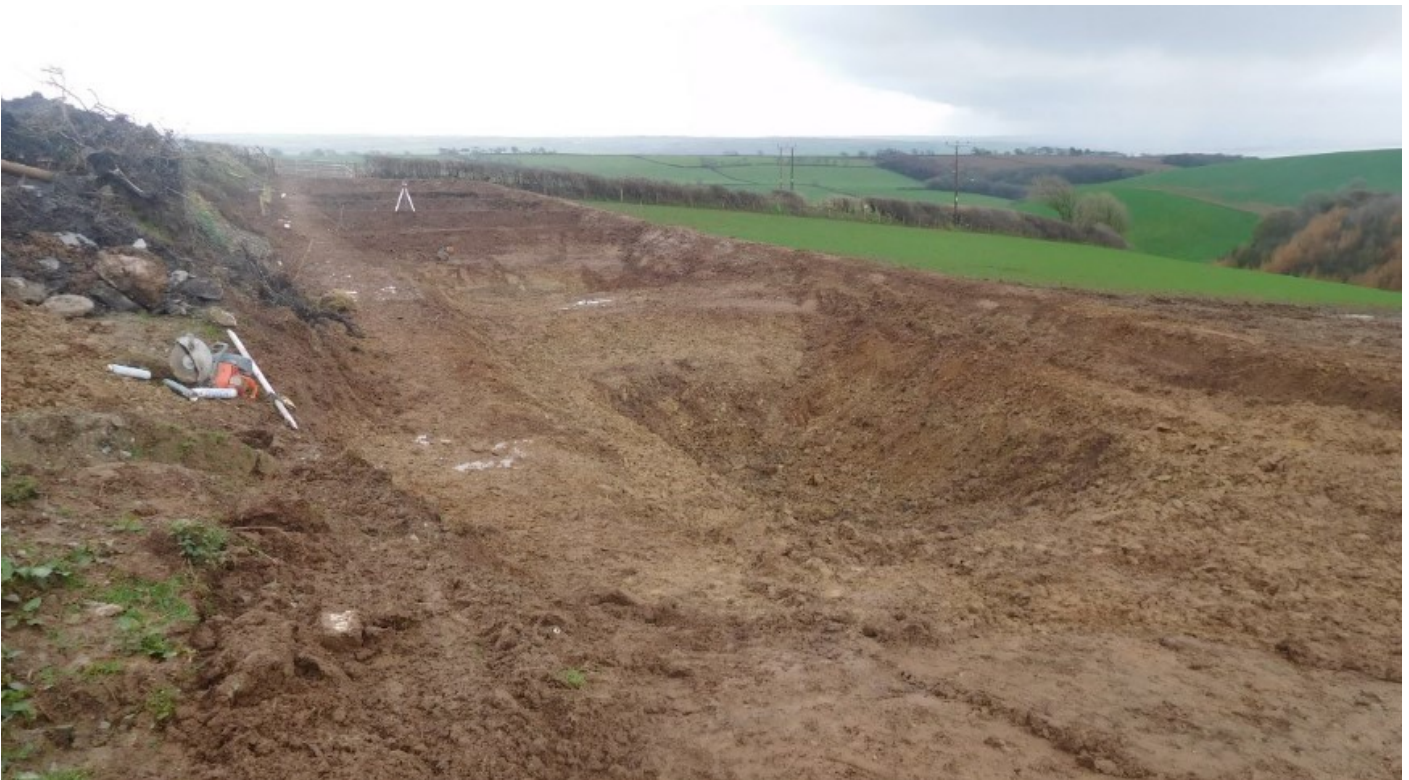
The 5 ponds mid-construction. Getting the levels right was a feat in itself.
