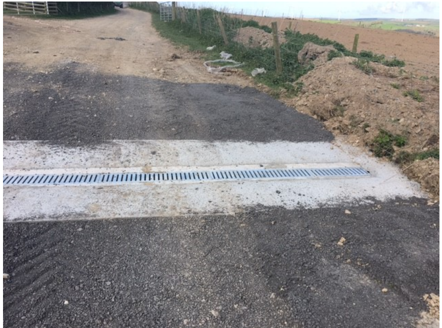
The cross drain at the bottom of the track. Water is piped from this into the ponds.
