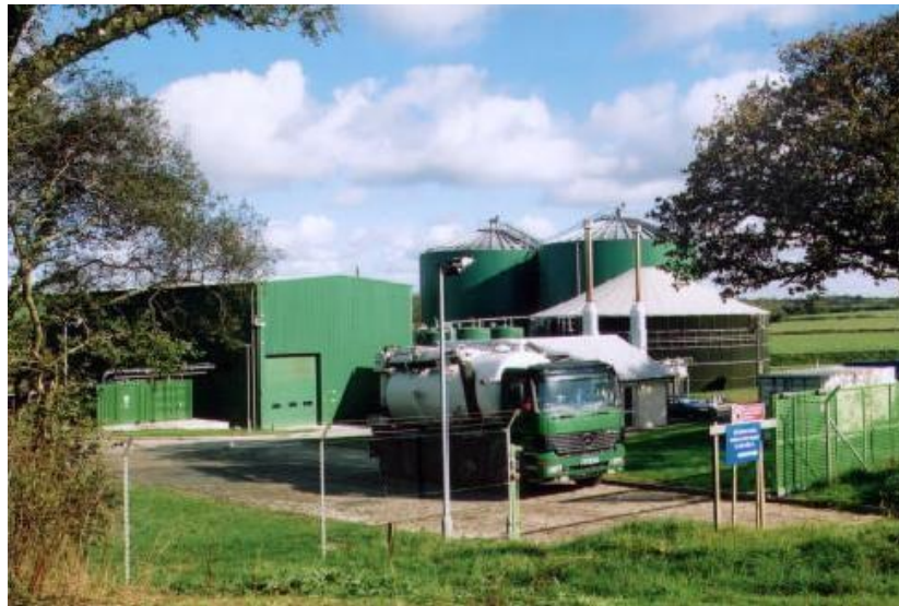
Andigestion Biogas Plant, Holsworthy
