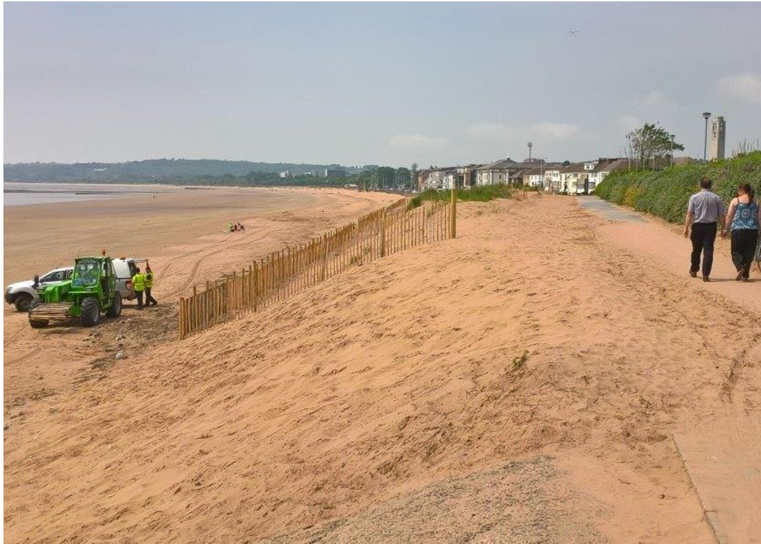
Figure 2 Installation of chestnut fencing to trap sand at Swansea Bay
