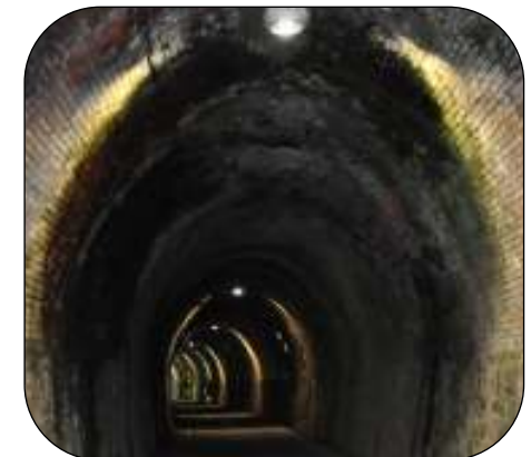
New LED lights at Landcross.
