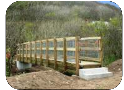
The new bridge at Mouth Mill.
