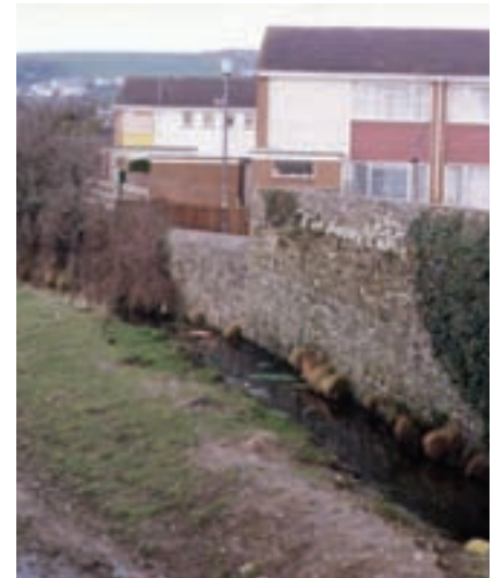
THE OLD SEA WALL AT WRAFTON
