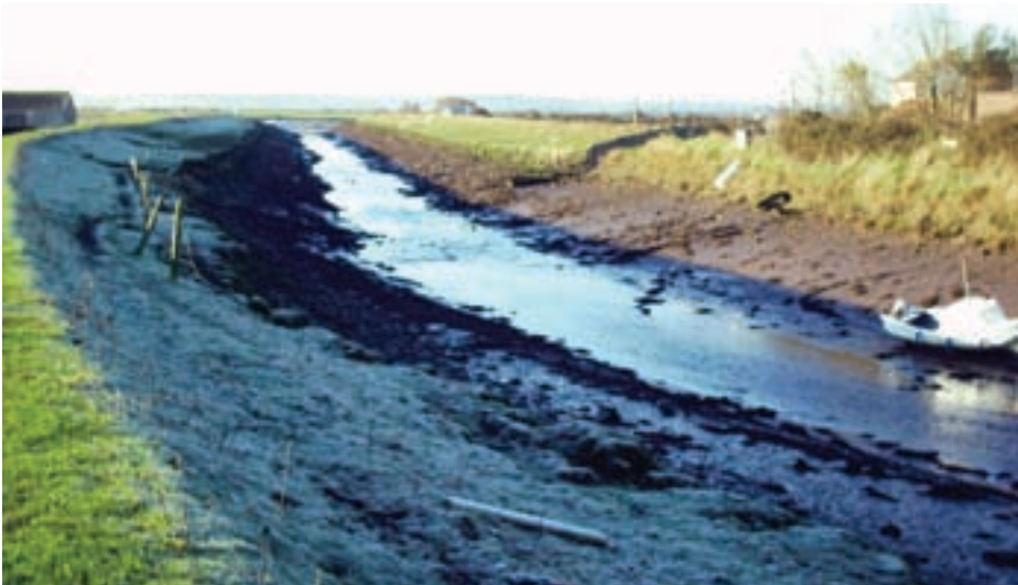
THE STRAIGHTENED SECTION OF THE BRAUNTON PILL, ALSO KNOWN AS THE 'NEW CUT'
