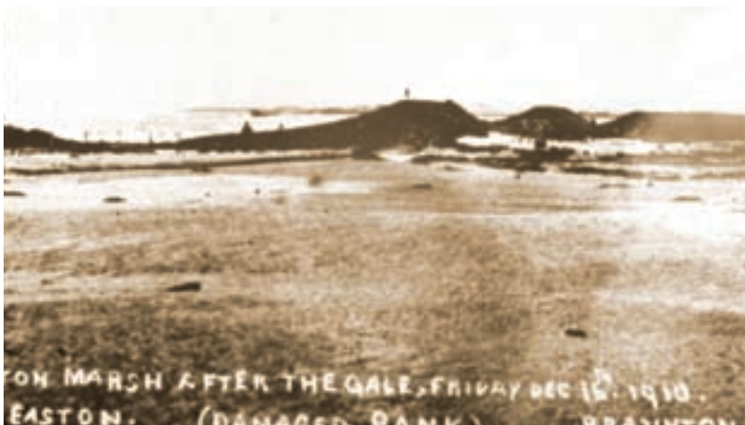
'BRAUNTON MARSH AFTER THE GALE - (DAMAGED BANK) 3
